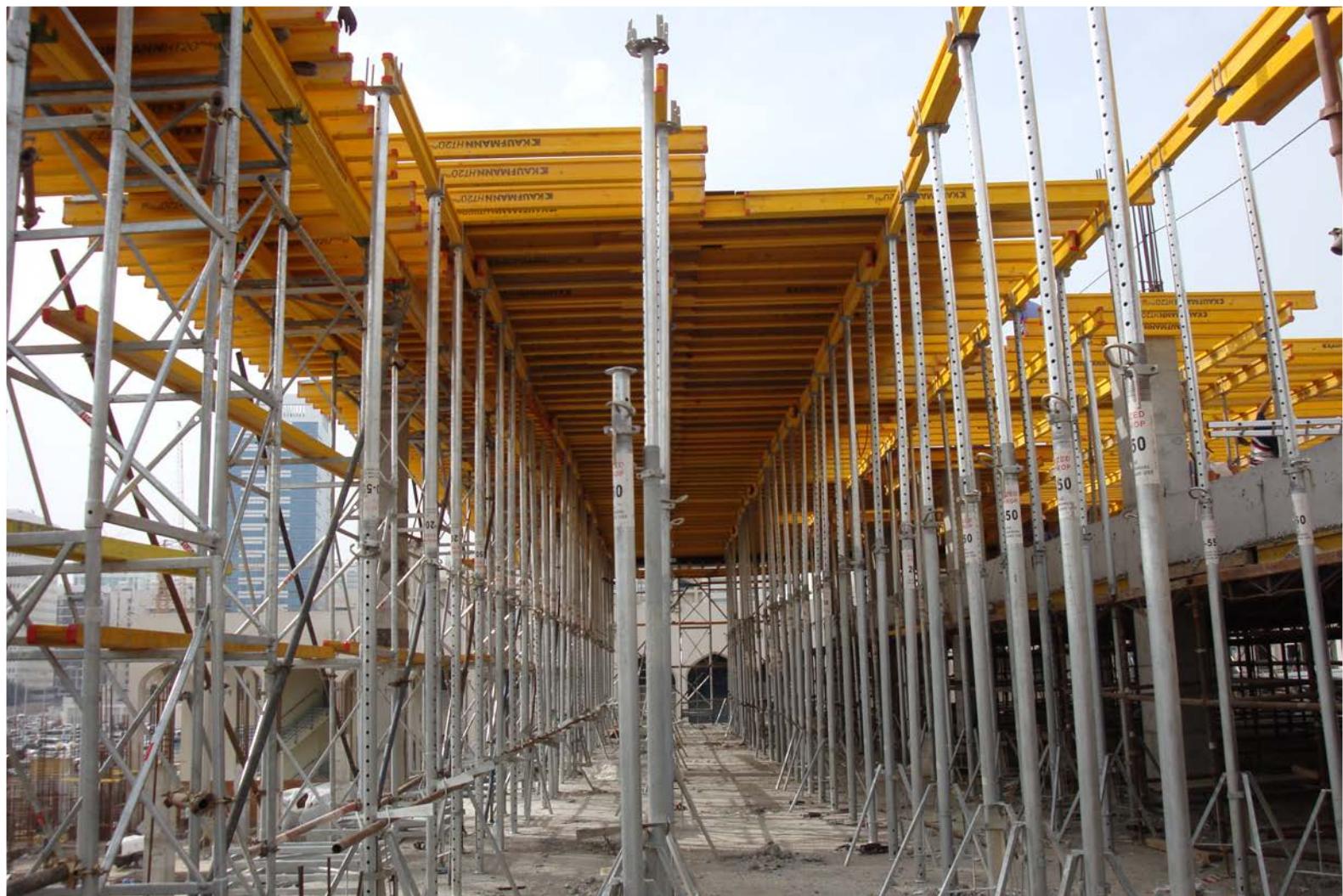
Using Slab flex @ maximum height (5.50m )
