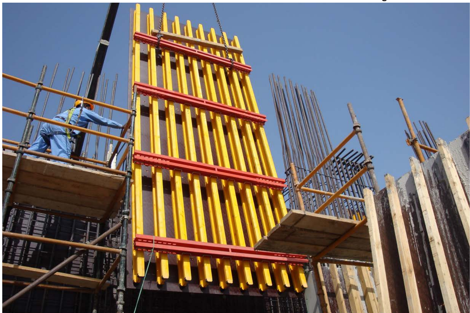
Erecting H20 panel for core-wall formwork setting-out
