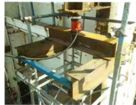
Photo 2 Load test arrangement
